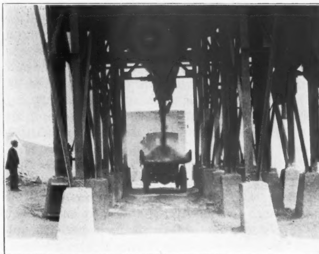
Loading a Truck
